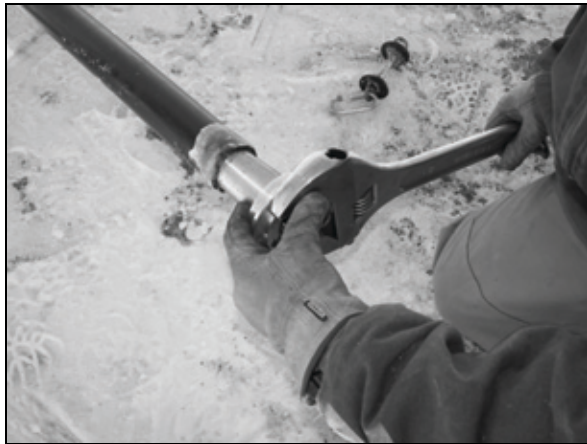
Figure 3 Place Threaded Adapter into Duct
