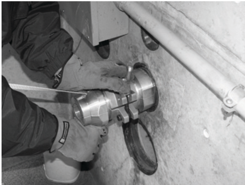
Figure 10 Secure Speed Ball Handle
