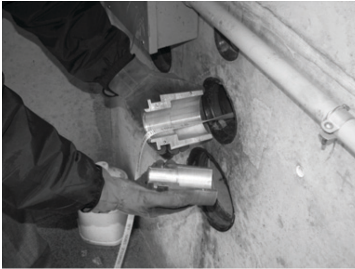
Fig. 7 Insert Threaded Adapter into Duct
