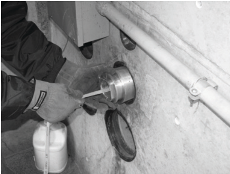
Fig. 8 Insert Threaded Adapter into Duct
