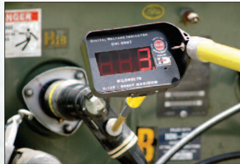
DVI-500T Measuring Elbow Test Point
